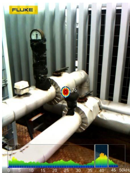
Leak detection on a pipeline
