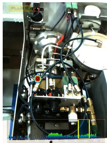
Air tightness inspection of complicated equipment pipelines
